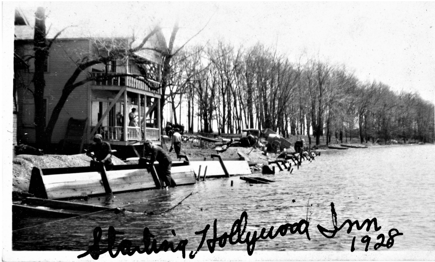
This photograph shows workers preparing to put in a concrete seawall. The cottage in the picture is believed to be the rental cottage that was later destroyed by fire. The main building and beach would be located in the area where the truck is parked.
